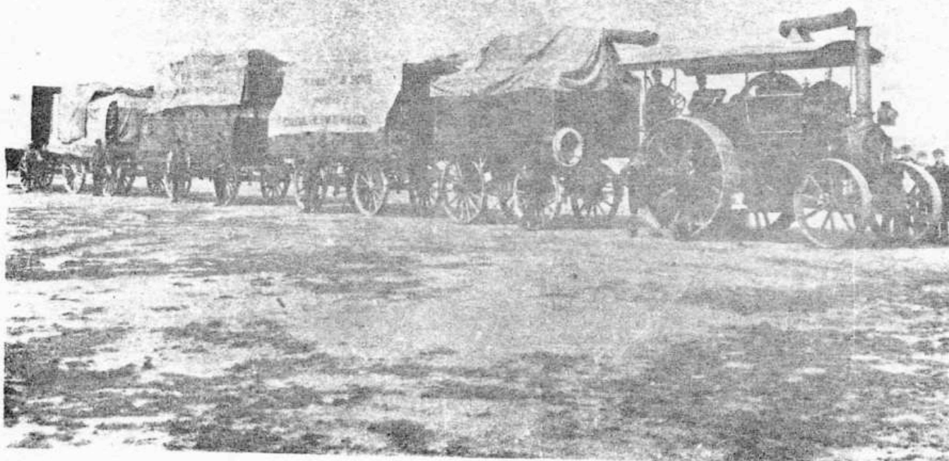
F. Bailey's Fowler no. 6926 with switchback loads.
